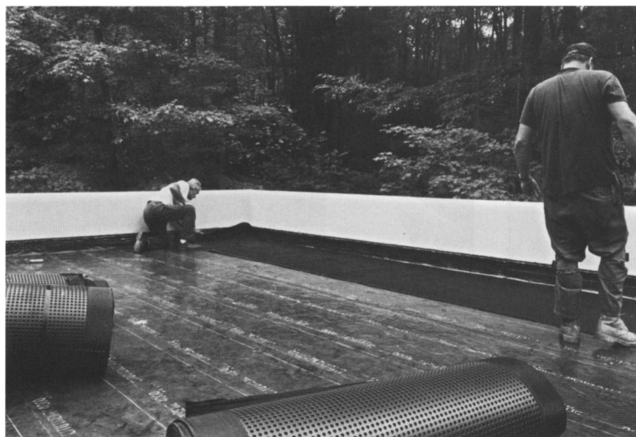
Fig. 7. Because the finished surface of the terraces consists of flagstones, the waterproofing is an IRMA (inverted-roofing-membrane assembly) system. Drainage mat was laid over the three-ply waterproofing on the master-bedroom terrace.
