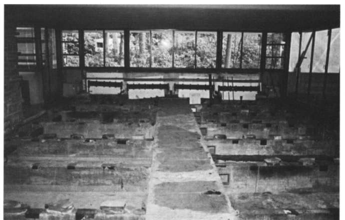
Fig. 6. The preeminent room of the house, the living room, was dismantled and the floor removed in order to grout the cracks in the cantilever beams prior to post-tensioning. One of the four main cantilever beams is visible at the center of the photograph, with concrete joists abutting it to either side.
